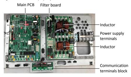
Figure 5-1.4: 20-32HP bottom layer of electric control box
